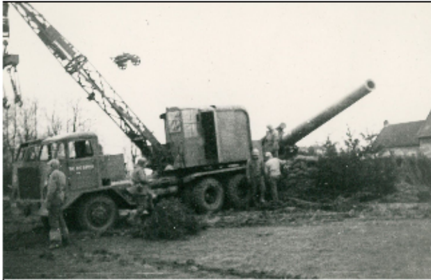
A crane ready to remove a tube
